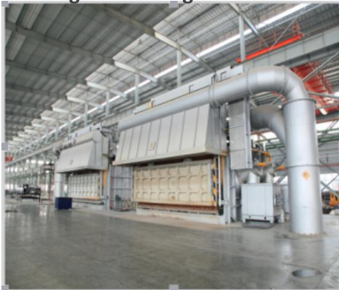
Melting and Casting
